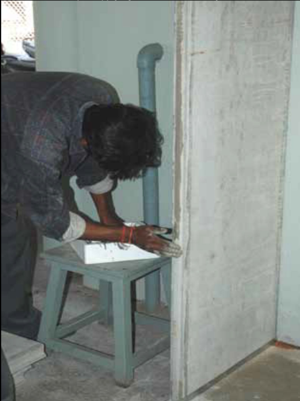
Step 4 : Applying Sodium Silicate & Fly Ash
