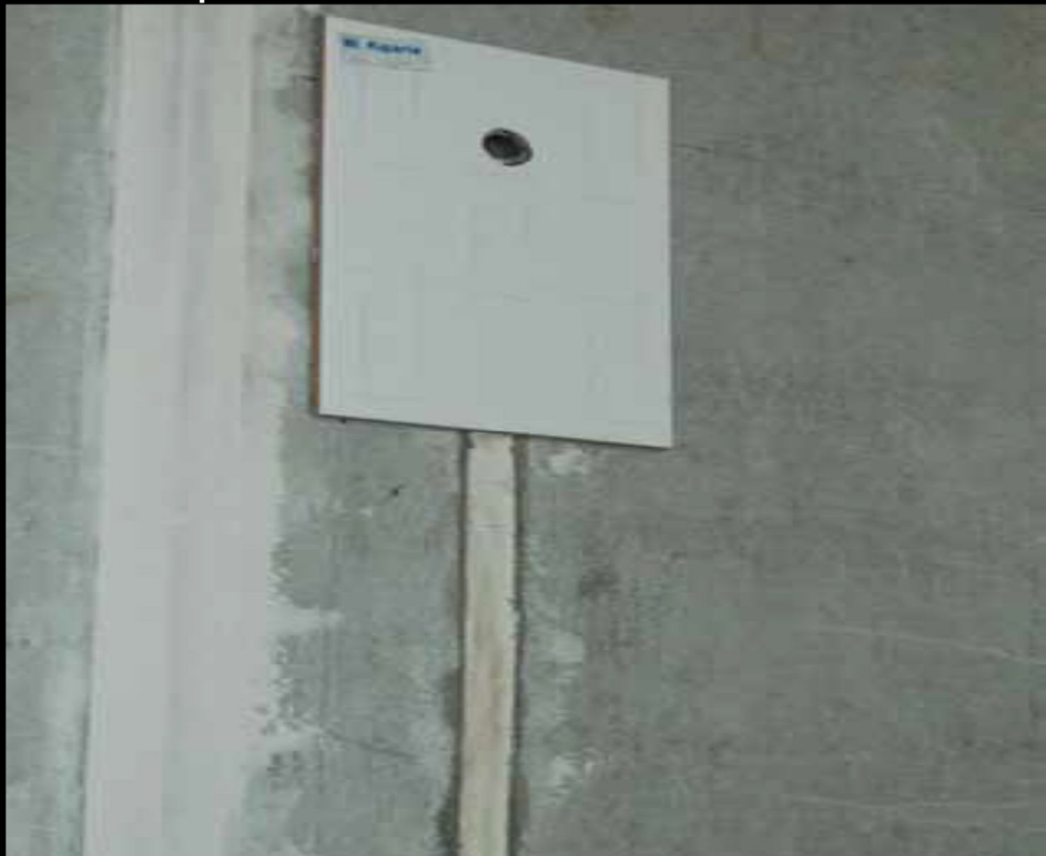
Step 8 : Tiles To Be Placed After The Service Lines
