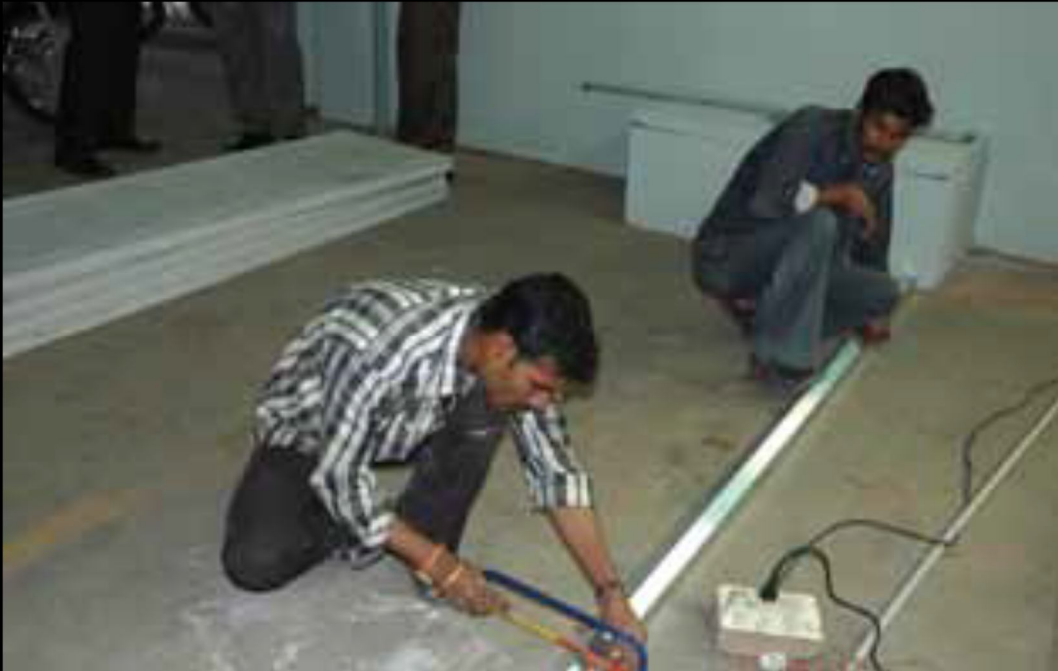
Step 1 : Marking Of Floor Channel
