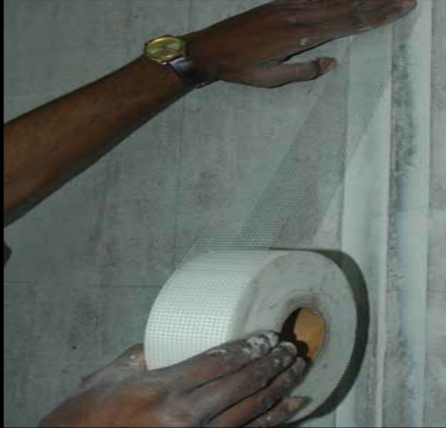
Step 5 : Filling Acrylic Putty & Applying Fibre Mesh Tape
