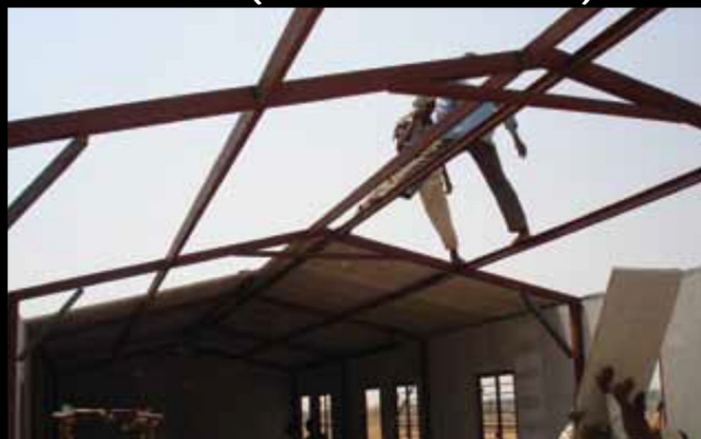
STEP 04 (PANELS OVER ROOF)
