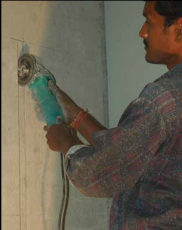
Step 6 : Cutting For Conduiting (Concealed Wiring)
